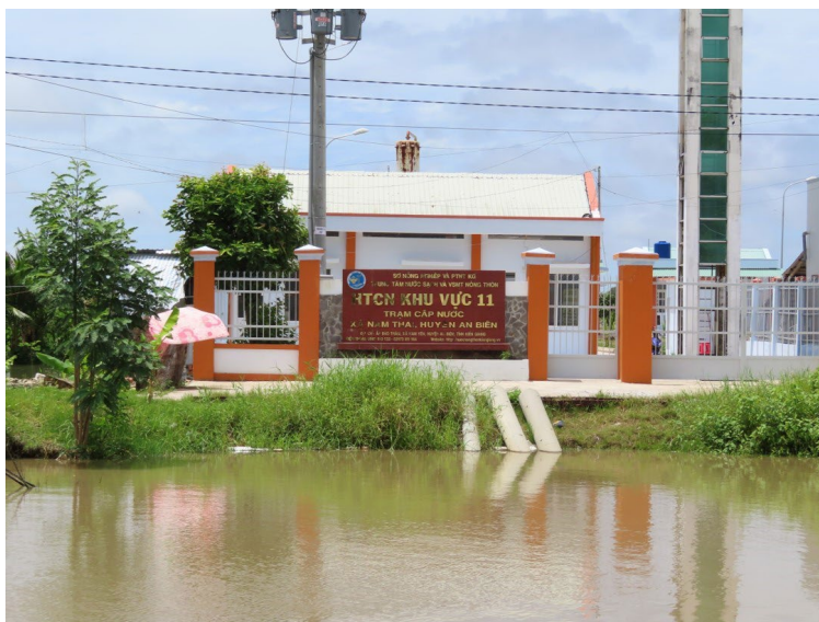
Figure 24. New water treatment plant on a Mekong River tributary. The goal is to supply treated river water to the villagers rather than potentially polluted and arsenic rich Mekong groundwater previously available via individual tube wells. Reprinted with the permission of the editor of the Open Journal of Soil Science.
