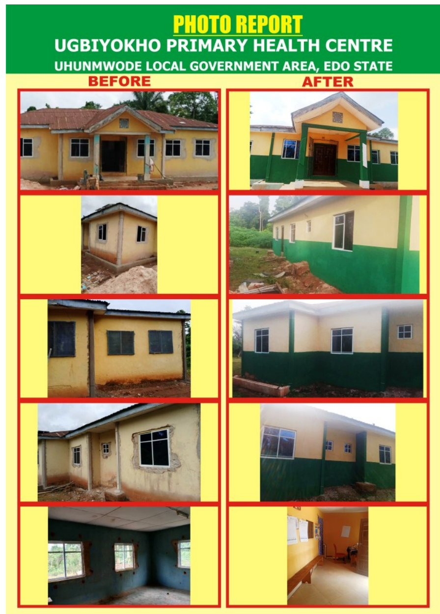
Figure A1. Infrastructure rehabilitation of Ugbiyokho Community Primary Health Center, Uhunmwode Local Government Area, Edo State, Nigeria. Representative before-and-after photographs demonstrate improvements implemented through the NANNNA Adopt-A-Primary Health Center (Adopt-A-PHC) Initiative, including facility renovation, exterior refurbishment, replacement of windows and doors, environmental improvements, and upgrading of interior clinical spaces to support safer and more functional primary health care service delivery.
