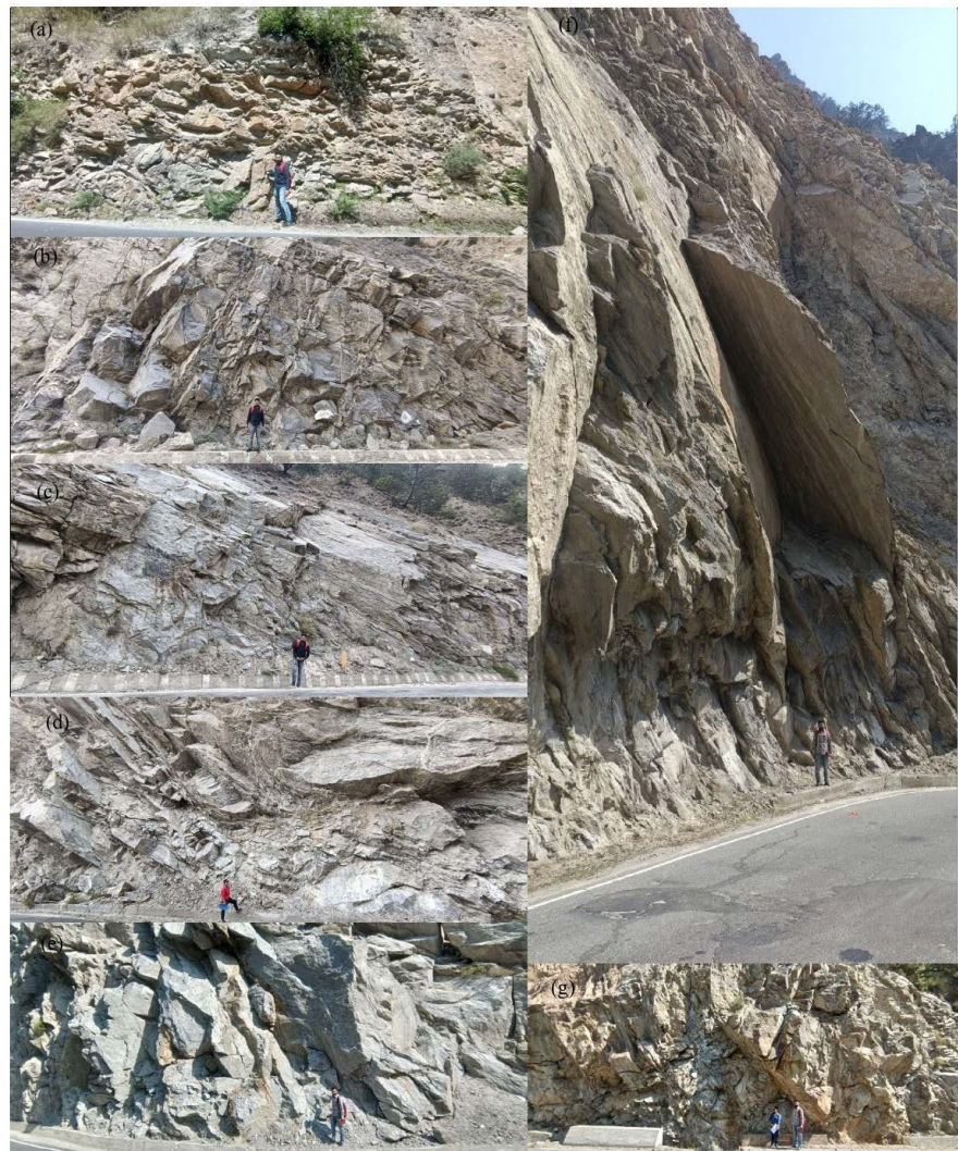
Figure 3. Field photograph of studied slopes: (a) S-1 jointed rock mass of gneiss. (b) S-2 jointed gneiss rock mass type. (c) S-3 planar failure in gneiss rock type. (d) S-4 wedge failure in jointed gneiss rock mass type. (e) S-5 wedge failure in gneiss rock mass. (f) S-6 shows wedge failure in granite-gneiss rock mass type. (g) S-7 planar and wedge failure in granite-gneiss rock mass.
