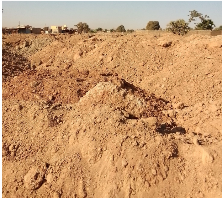
Figure A1. One of four (4) disposal sites for materials excavated from the road construction site.
