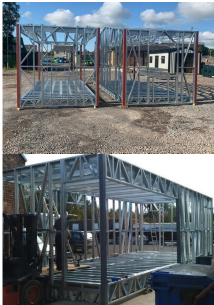
Figure 18. Typical light gauge modular units (Used with permission) ( https://ccssteelframing.com/modular-building/ ) [Site visited 06/21/26].
