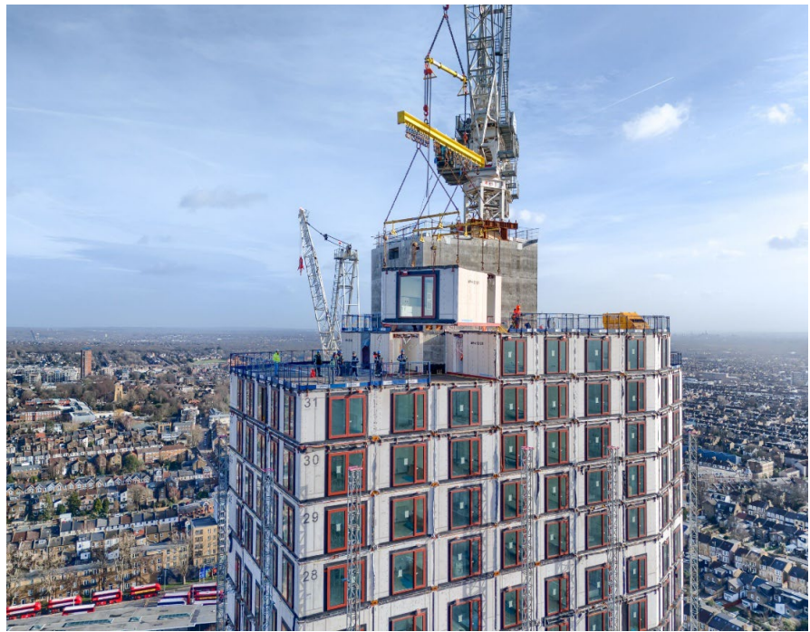
Figure 13. Roof mount crane to lift modular units in highrise modular construction (Used with permission. Credit for the image: Britlift, Apex Drone Photography, and Outpost Management: https://britlift.com/lifting-modular-homes/ ) [Site visited 06/21/26].
