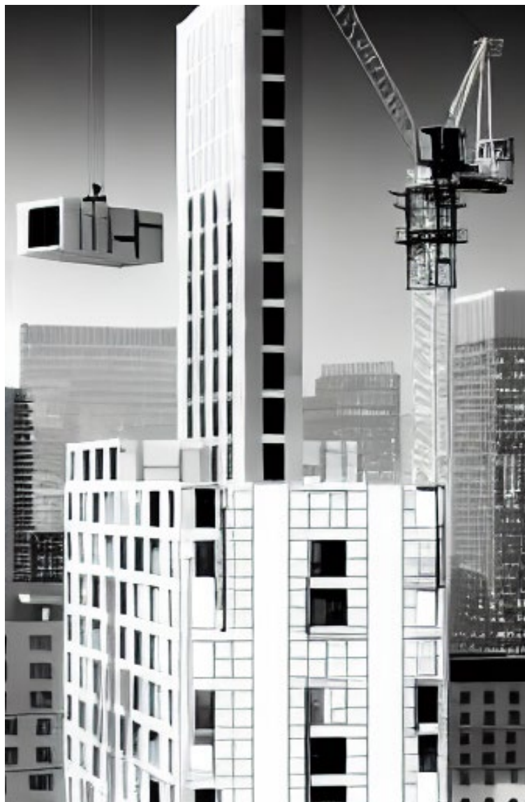
Figure 8. Modular units being stacked on top of one another to form a high-rise building (Adapted from [23]).
