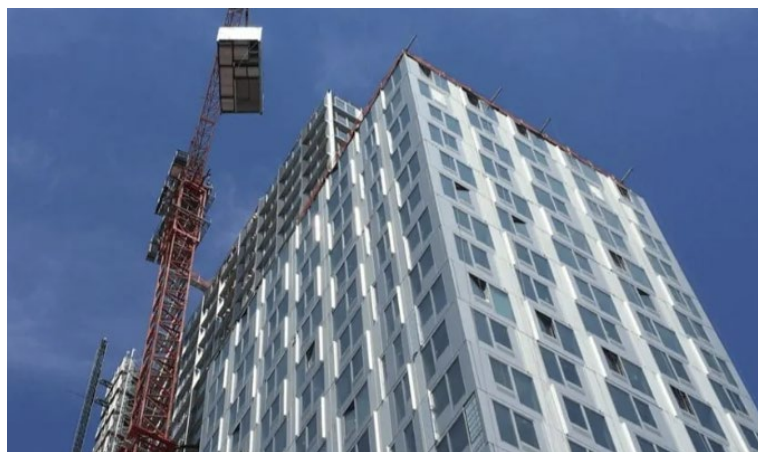
Figure 4. Example high-rise modular construction (Used with permission) https://s3da-design.com/steel-framed-modular-construction-for-high-rise-hotels-what-you-need-to-know/ [Site visited 06/20/26].
