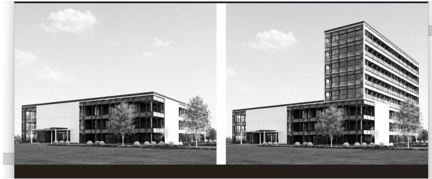
Figure 9. Conceptual vertical expansion example: (left) preexisting structure; and (right) modular expansion on top (Adapted from [23]).
