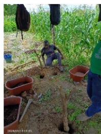
Installation of the brackets
