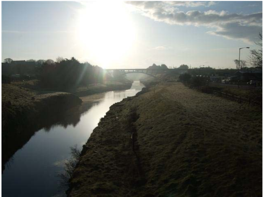
Figure 3. Cathleen's Falls Bridge taken from the Allingham Bridge (13/04/2008 am) [7].
