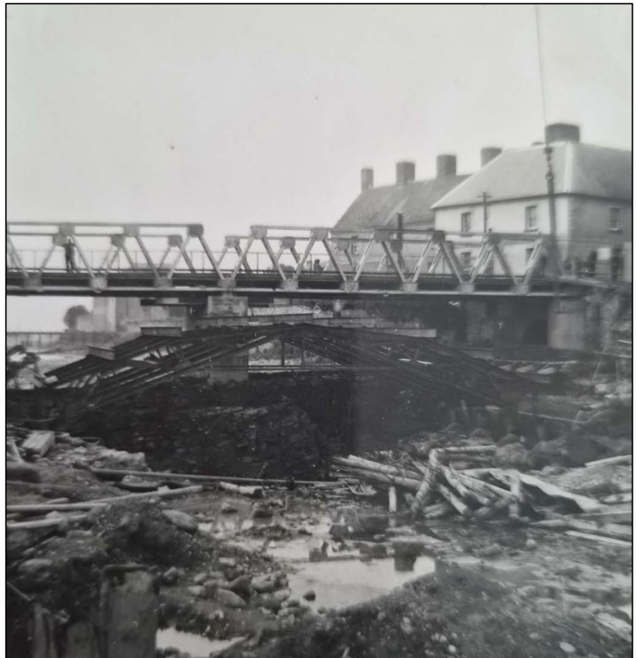
Figure 6. Allingham Bridge construction commencing (04/09/1946) [10].
