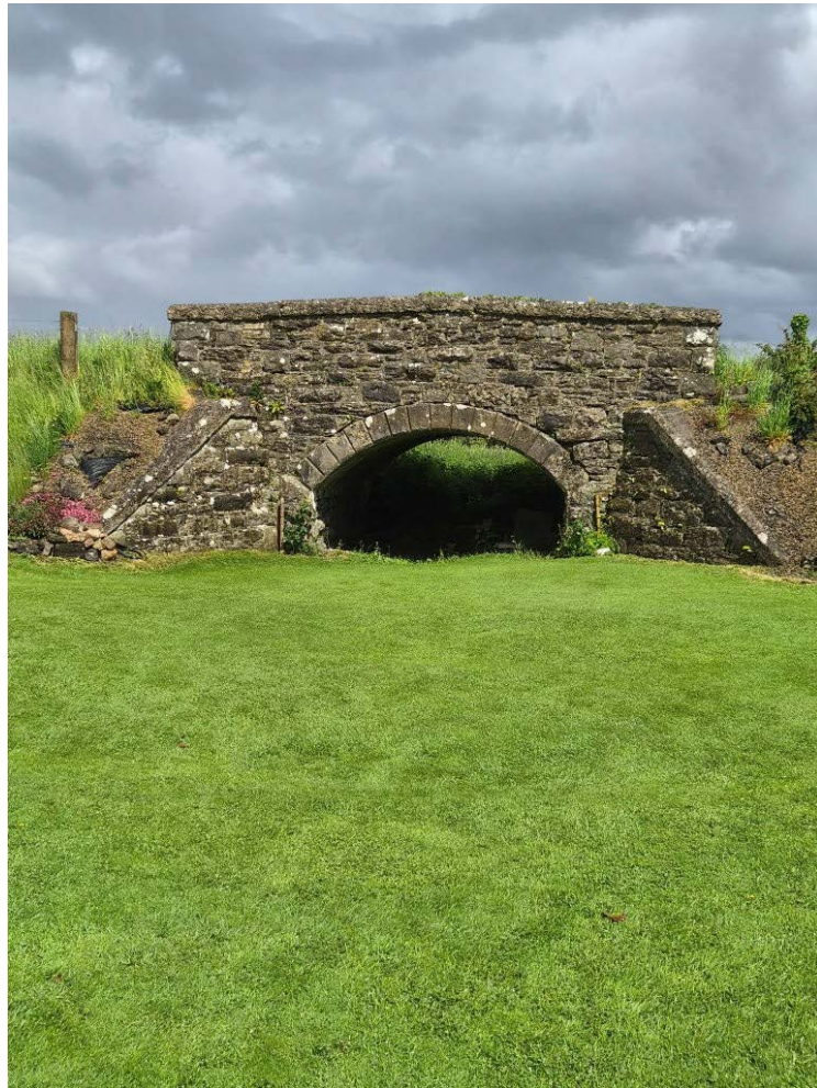
Figure 11. Abandoned CDR Bridge in Private Garden (08/06/2026) [22].
