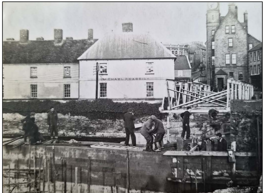
Figure 4. Temporary bridge under construction (06/01/1946) [8].
