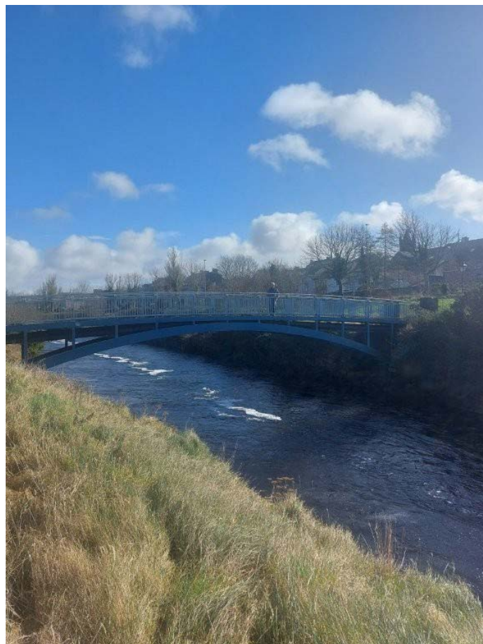
Figure 2. The Millennium Footbridge from downstream (02/03/26) [6].
