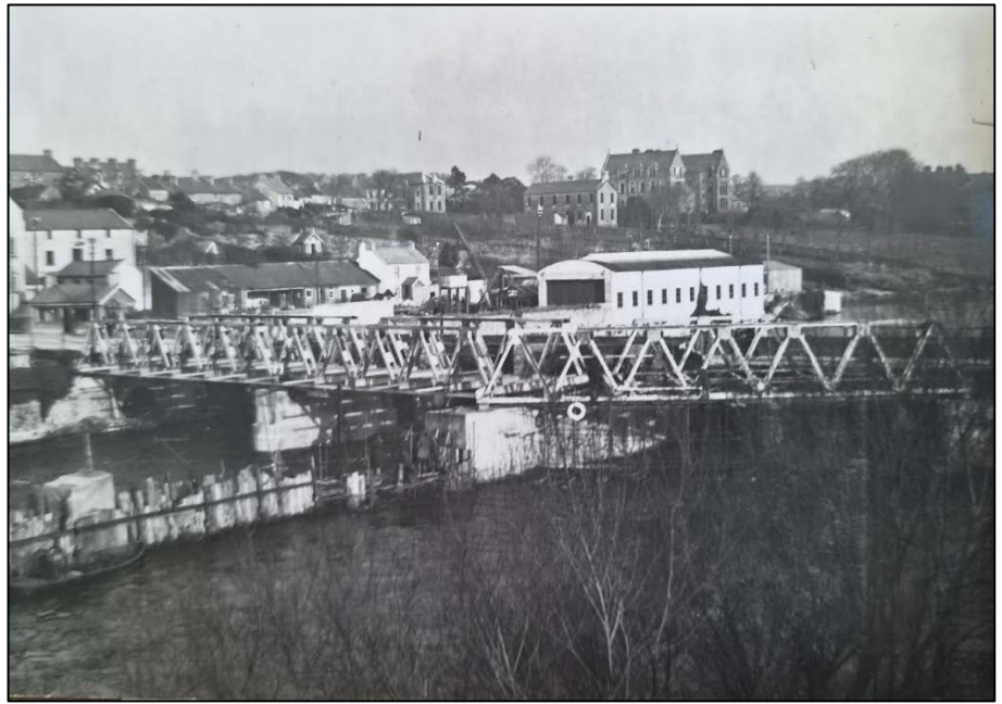
Figure 5. Temporary bridge constructed (19/01/1946) [9].
