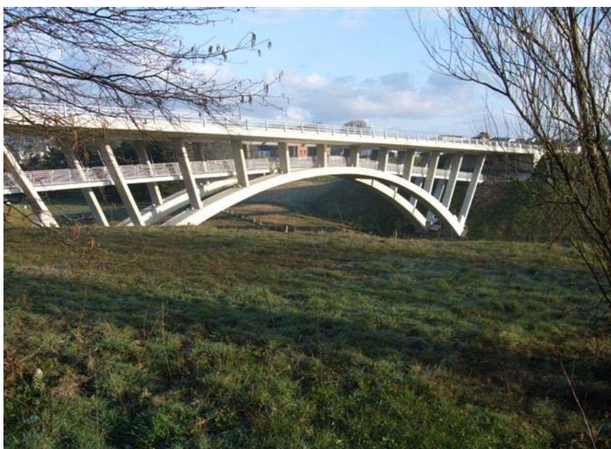
Figure 10. Cathleen's Falls Bridge from downstream (13/04/2008 pm) [17].
