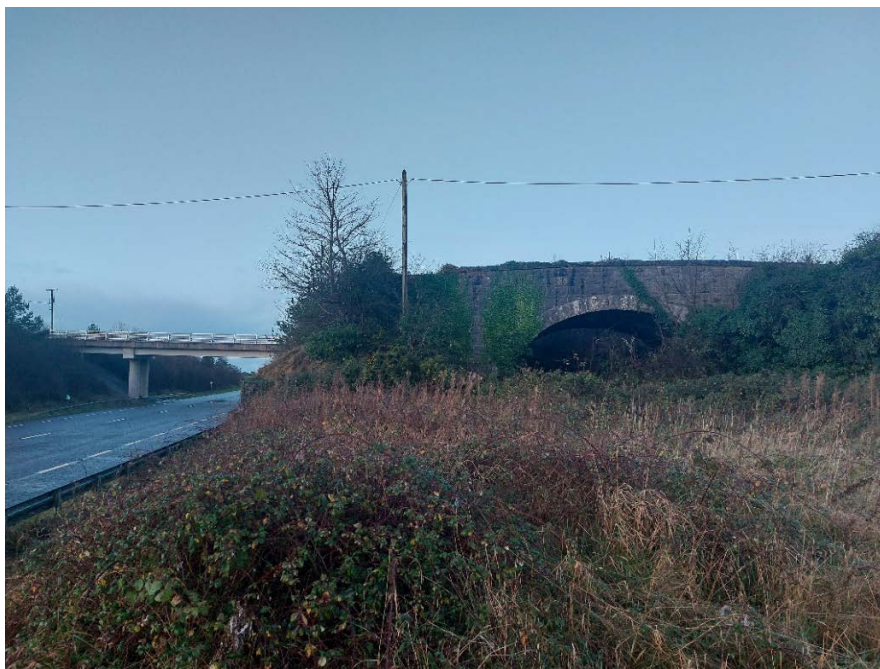
Figure 14. Abandoned GNR Bridge beside the N15 Road (08/06/2026) [25].
