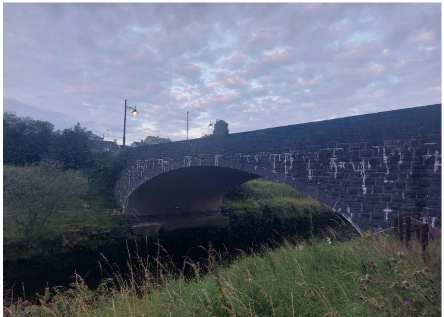
Figure 8. Allingham Bridge from upstream (27/07/2025) [12].
