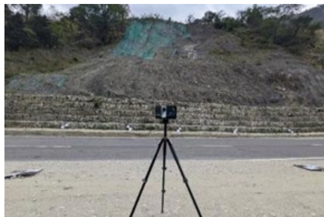
Figure 2. Scanning by FARO S350+ of Kshetrapal landslide.
