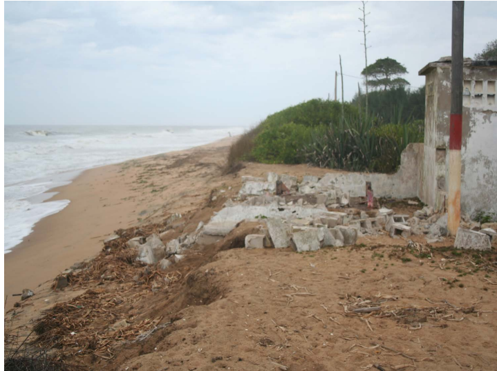
Figure 12. Erosion slope 50 m from.
