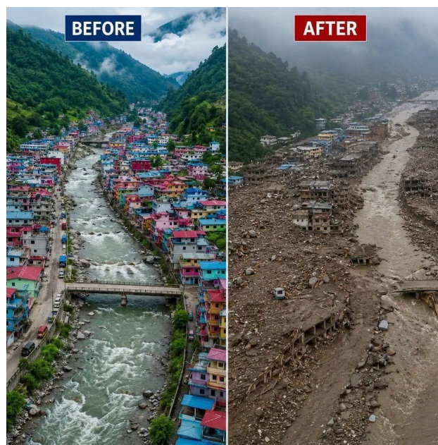
Figure 4. Rasuwa Bazaar before and after the August 26, 2026 flood.
