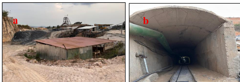
Figure 3. Underground ASM sites at Dompase showing (a) Underground Mine Set-up (b) A Typical Inclined Tunnel.
