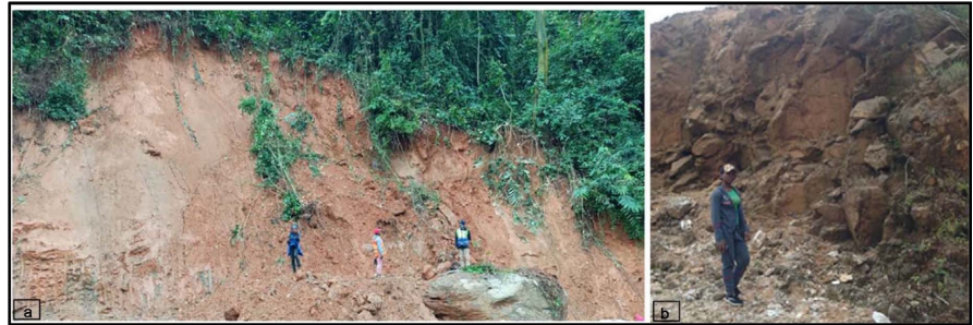
Figure 1. Overview of some vulnerable sites on the SWEBP. (a) Risk of rotational landslide; (b) rockfall risk2-Laboratory methods.
