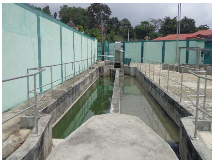
Figure 1. Blockauss pumping station.
