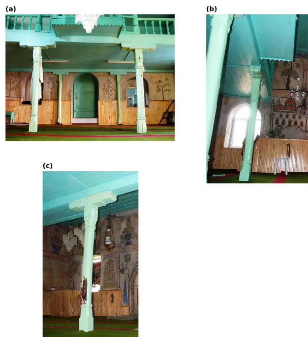
Figure 9. Gallery floor and wooden columns (Sedes, 2016).
