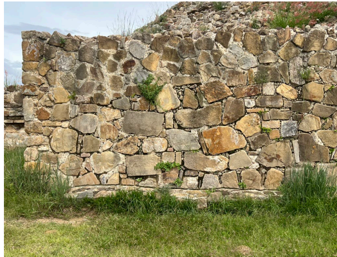
Figure 17. Building “G”, west side (Author’s photograph).
