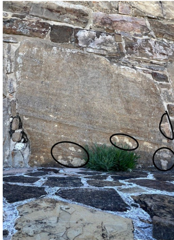
Figure 14. Stucco remnant on a slab of Building “J”, north-west side (Author’s photograph and enhancement).
