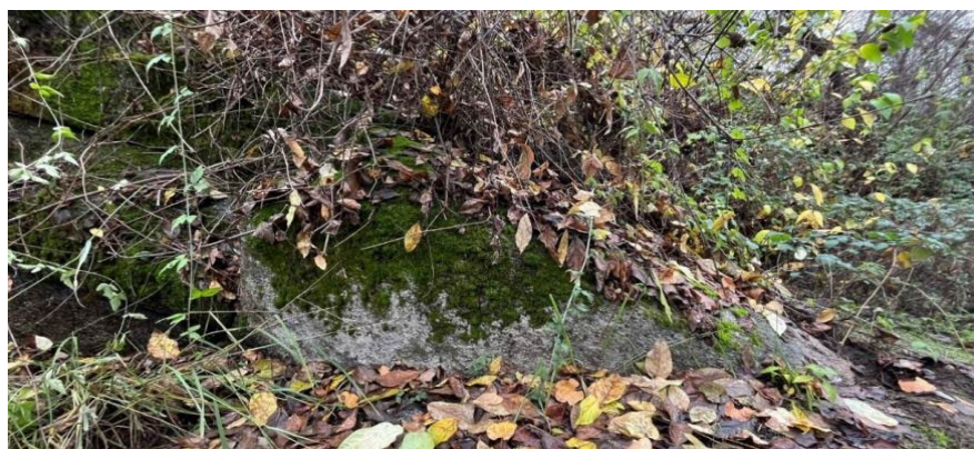
Figure 2. Close-range view of the same exposure showing joint planarity and course boundaries. Photograph: Gary Bruce.
