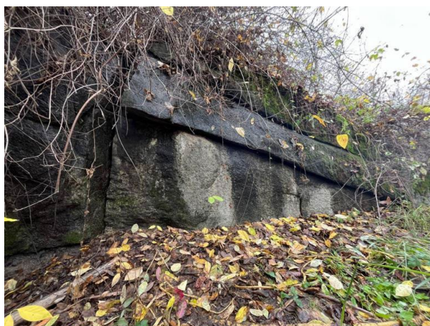
Figure 1. Coursed granite exposure showing laterally continuous, roughly rectangular blocks separated by planar joint surfaces, Three Rivers, California. Photograph: Gary Bruce.
