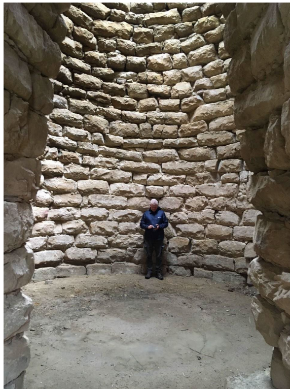
Figure 15. Interior corbelled dry-stone construction inside a nuraghe, Sardinia, Italy, showing coursed masonry technique.
