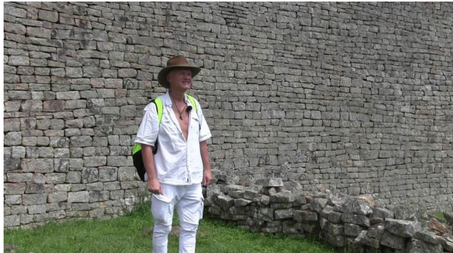
Figure 16. Great Zimbabwe, Masvingo Province, Zimbabwe: coursed dry-stone granite wall of the Great Enclosure, with a person for scale.
