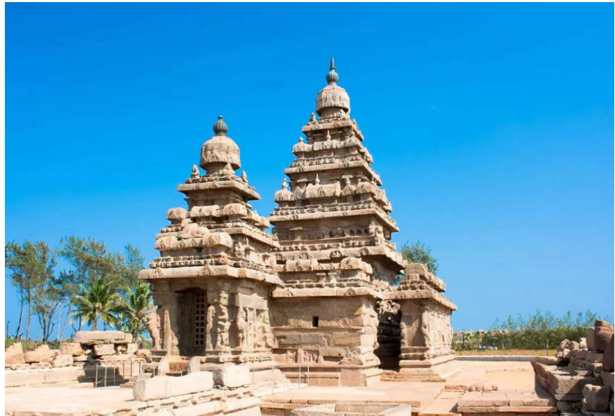
Figure 23. The Shore Temple, Mahabalipuram, Tamil Nadu, India: a granite structure carved and assembled directly on a coastal granite outcrop.
