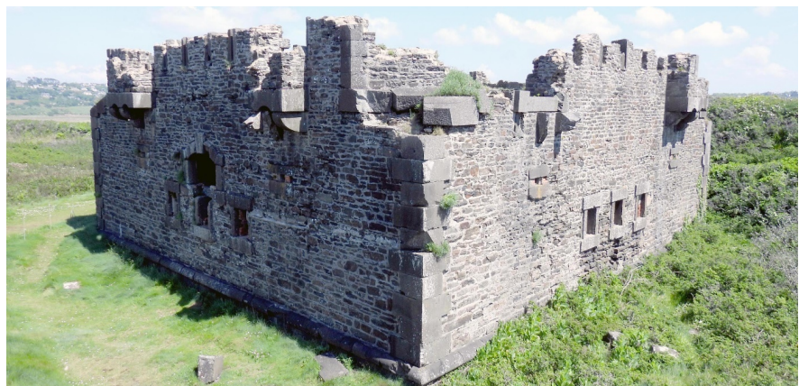
Figure 8. Fort de l'Aber (1), North-East view.
