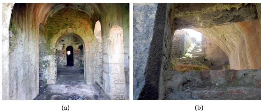
Figure 9. Fort de l'Aber—(a) internal corridor, on the right access portal to the coverage ascending stair; (b) coverage ascending stair.
